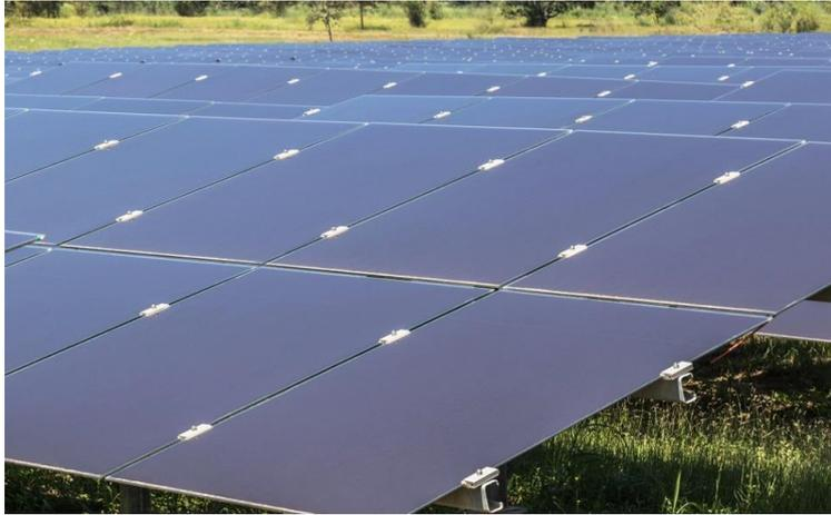
**Figure 1.6:** Cadmium Telluride photovoltaic cells.
